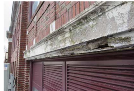
View of pronounced stone cladding deterioration as seen at north facing elevation of original building—also note exposed and corroded reinforcing steel
