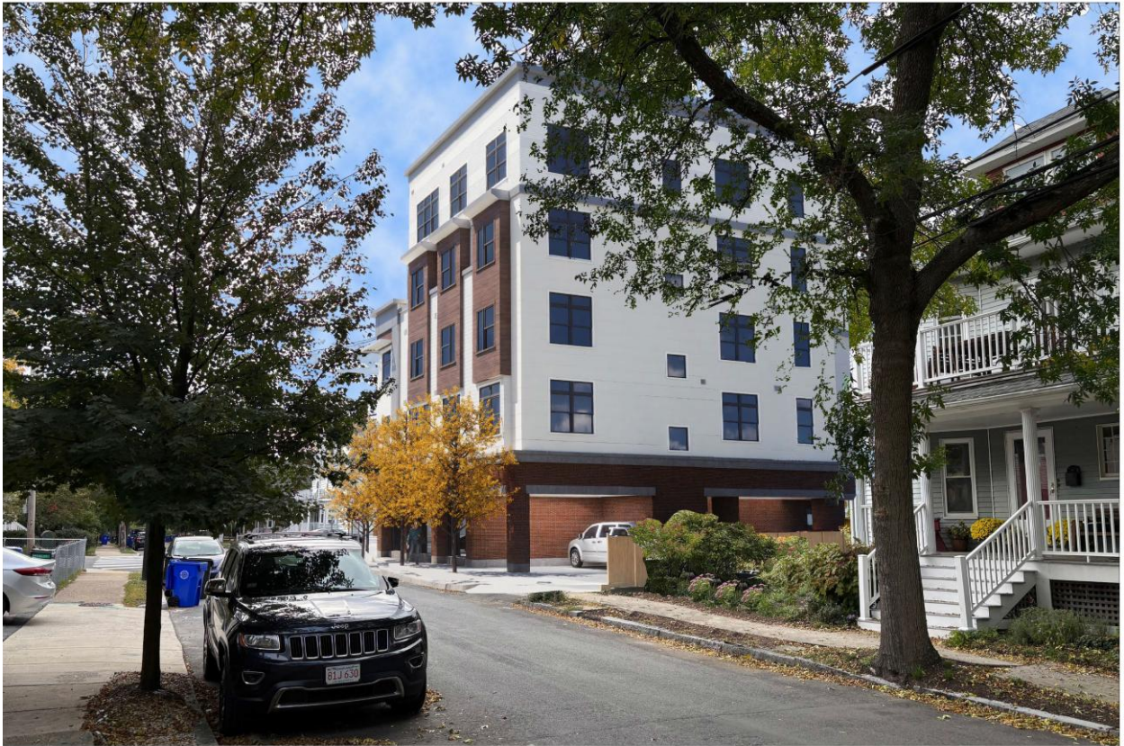
The open area at street level under the building's second floor, with part of a white car showing, is the platform parking area.
